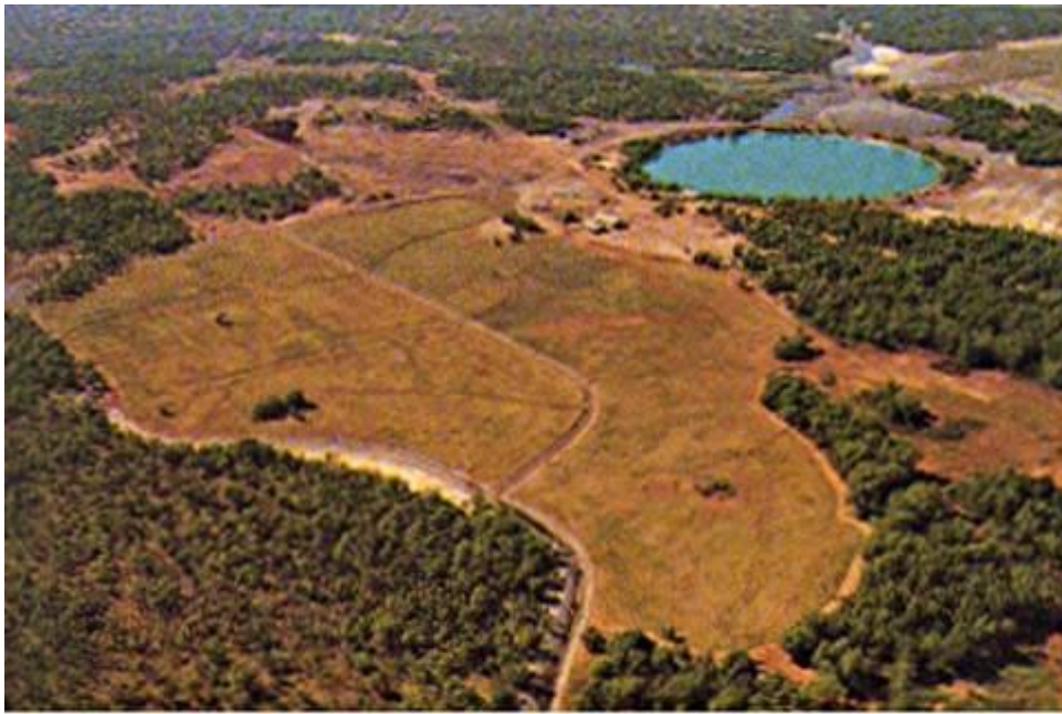
Aerial view of old tailings dam after rehabilitation, May 1986.
