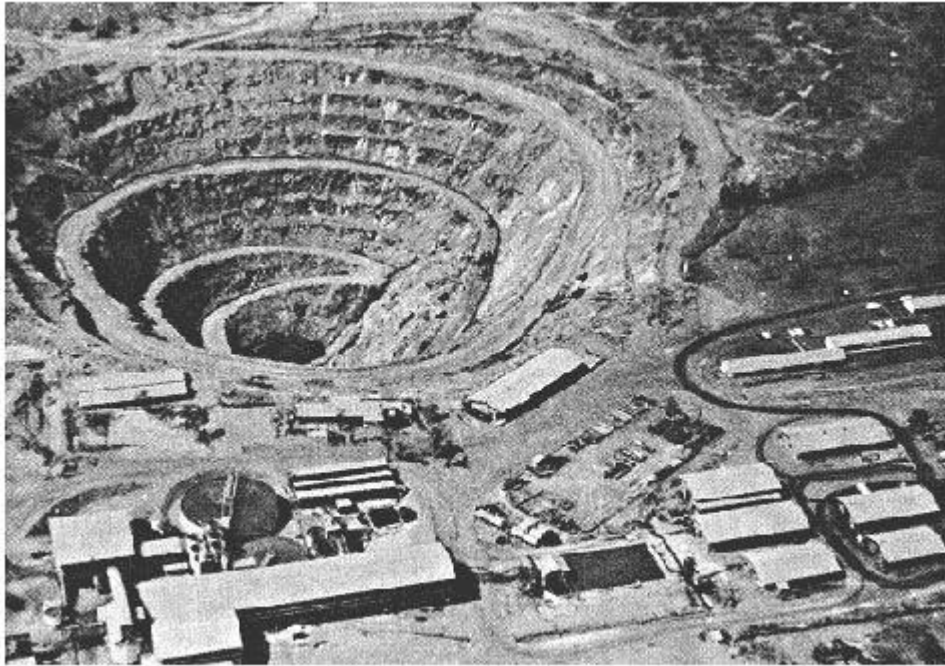
White's Open Cut and Rum Jungle treatment Plant, during the late 1960's. Completed to a depth of 350 feet in 1958.
