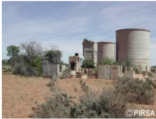
Treatment building and headframe c.1955
