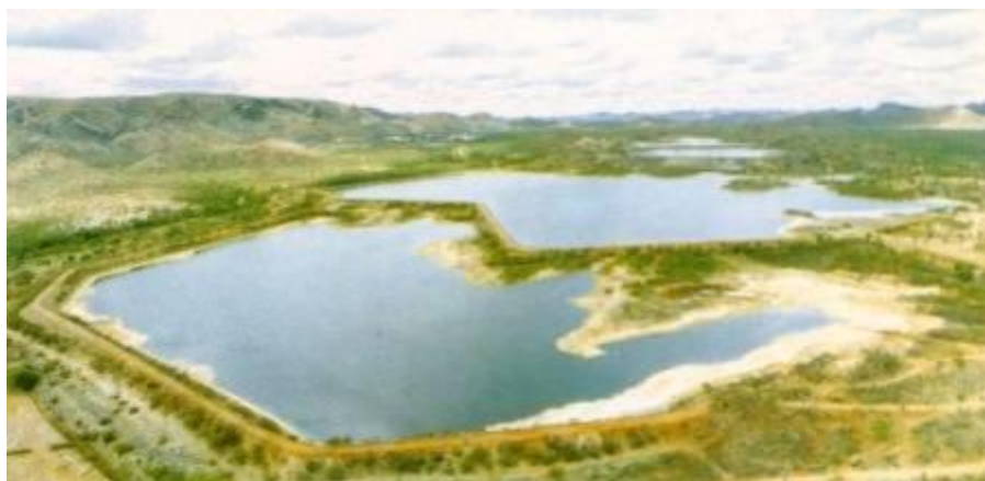
Aerial view of the tailings dam and evaporation pond, 1976-82.
