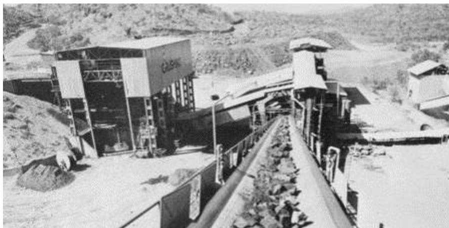
Crushed ore conveyor, second period of operation, 1976-82.
